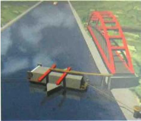
Shifting the deck on concrete beams.
